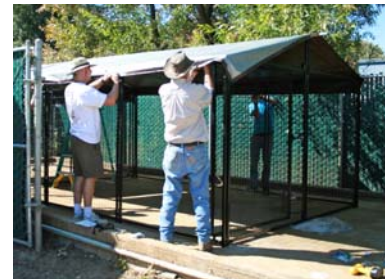
New fence panels for dog exercise area
